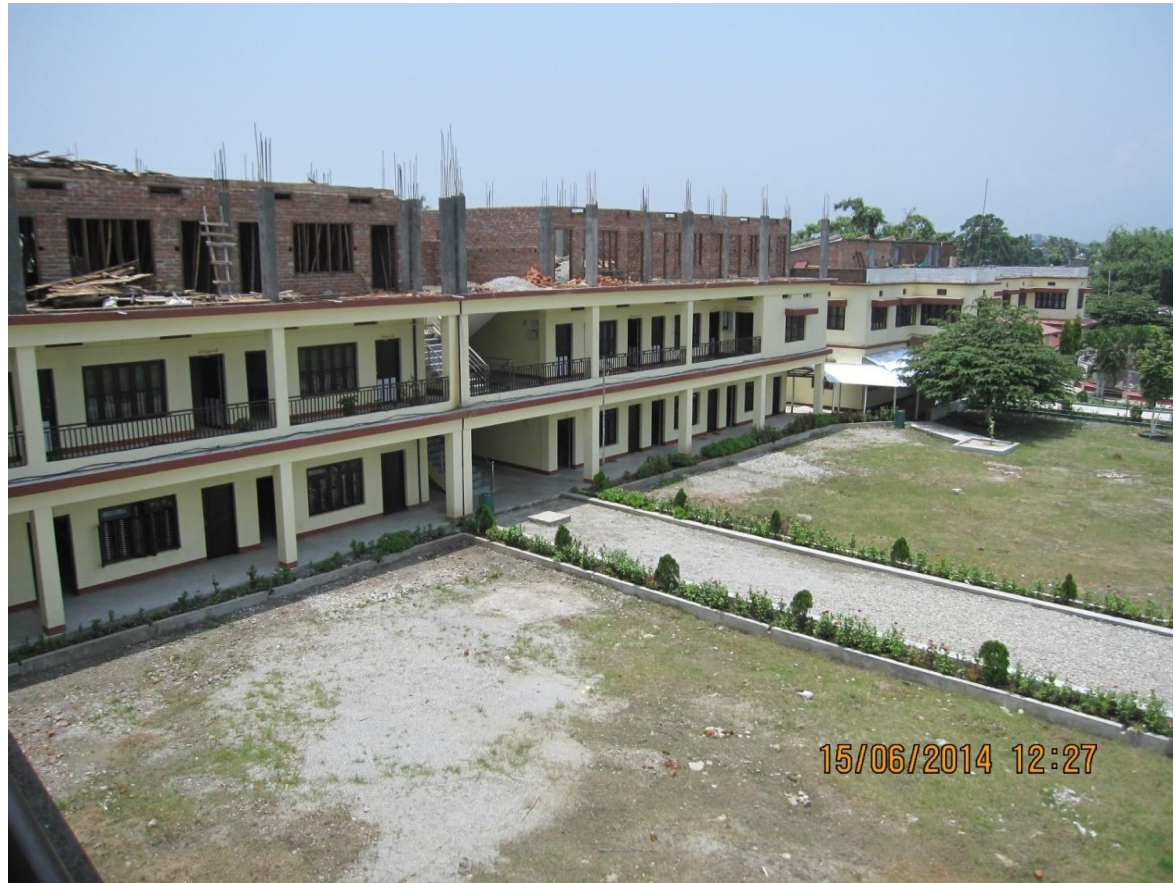
Figure 20: Science Building under construction
