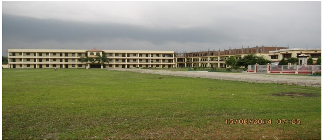
Figure 16: Administrative, Science and Teaching Building
