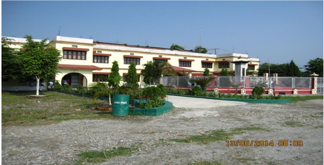
Figure 12: Existing Administrative Building
